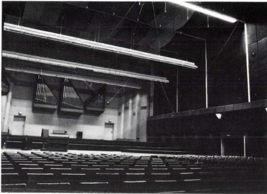
Fig. 9. The Hans Rosbaud Studio of the Südwestfunk broadcasting organization at Baden-Baden (Federal Republic of Germany). This studio has been provided with an MCR system of 70 channels. The microphones can be seen suspended from the ceiling; the loudspeakers are incorporated in the walls.
